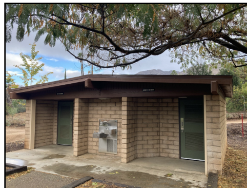
Repaired upper restrooms
