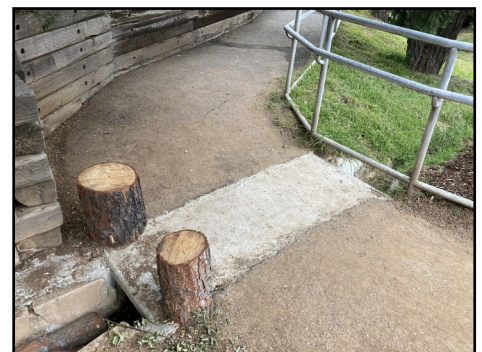
New culvert for better drainage
