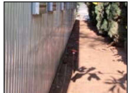
Channel drain outside the greenhouse
