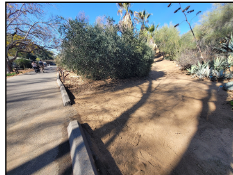
The new opening in the curb to access the Desert Garden
