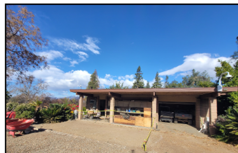
The location for the new storage bin
