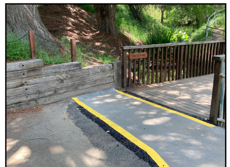
Asphalt repair by the Turtle Pond
