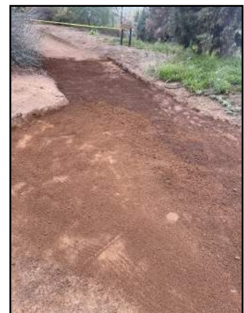
Perimeter trail repaired
