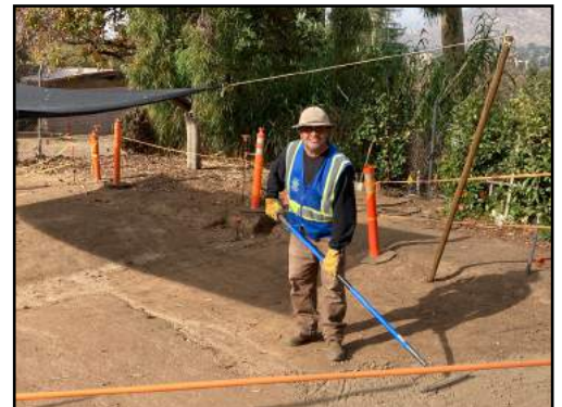
Jorge Fregoso working on the drainage outlet
