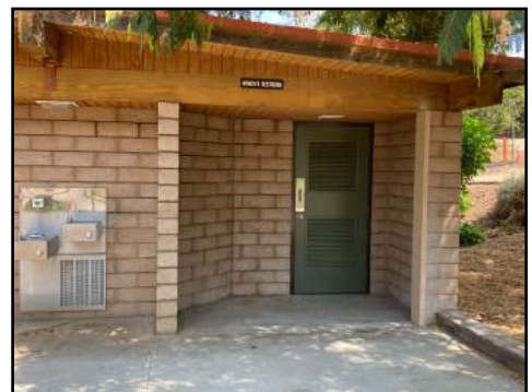
Restroom renovation completed
