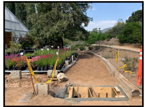
Drainage repairs near upper nursery
